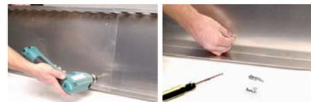
**Step B:** If BT-17S is required for your installation, see those instructions prior to continuing. Install "**Face Stiffener**" in the center of BB-ADJR or roughly over the center of the BT-17S location if used, and flush to the top of the BB-ADJR with the tab pointing down in the rear and up at the front. Mark and drill the two(2) 1/4" holes located at front and rear of Face Stiffener. Place remaining #12 x 1/2" screw in front hole and secure with nut.
